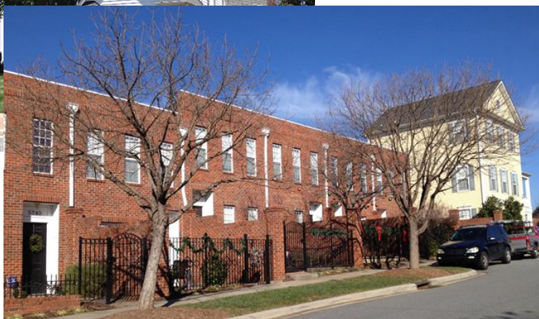
The photograph (left) is of a four-unit single-family attached town-house property in Kannapolis, North
